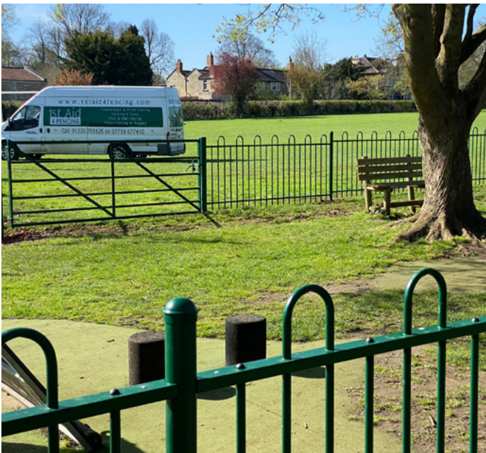
Anti Trap Bow Top fencing with 3.0m wide Metal Field gate in background
