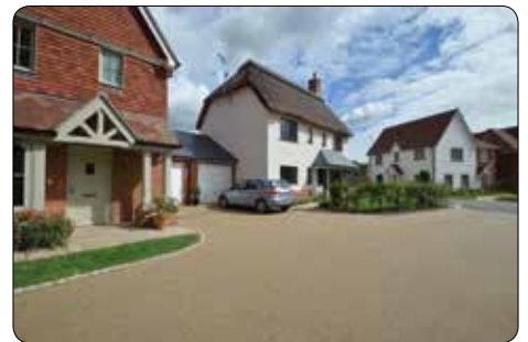
Berkeleys Homes: The Ashmiles, roadway and paths for new build homes, Barns Green, West Sussex.
