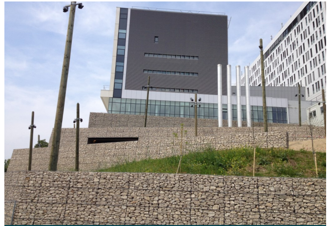
Figure 1: Example of Galmac C3 welded gabion application
