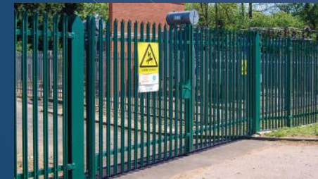
Palisade Fencing & Gates
