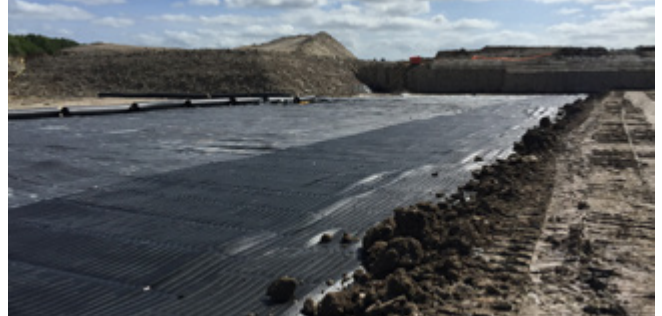
ParaLink® used over mine workings in the South West
