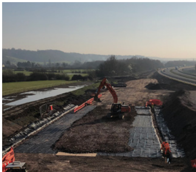
ParaLink® placed over soft soil on the M49, Bristol
