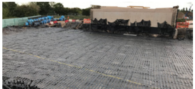
ParaLink® used over piles at Colley Lane, Somerset
