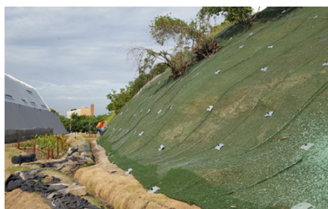
MacMat® R soil stabilisation in industrial park
