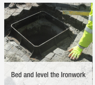
Place tuffset 60 on top of rebuilt brickwork/courses
