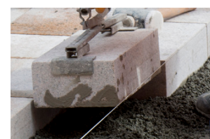
Lay mixed mortar onto the base and bed the paving unit
