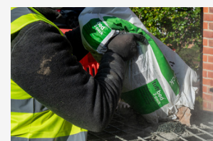
Mix binder and aggregate 1 binder : 4 aggregate
