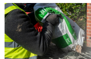
Mix binder and aggregate 1 binder : 4 aggregate
