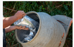
Mix binder and aggregate 1 binder sachet : 1 aggregate
