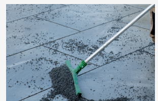
Squeegee tuffflow into the joints. Remove excess
