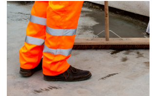
Clean the area
