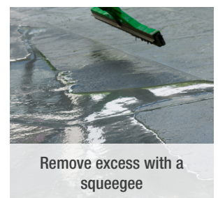
Pour tufftop onto surface and squeegee into joints
