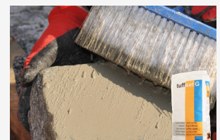
Apply tuffset G to concrete base and paving unit
