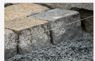
Lay mixed mortar onto the base and bed the paving unit
