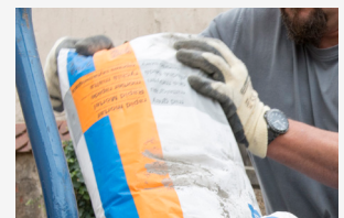
Mix binder and aggregate 1 binder : 2 aggregate
