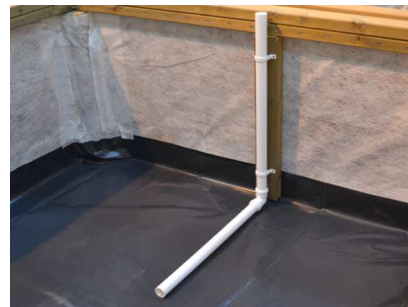
Polythene liner with filler pipe
