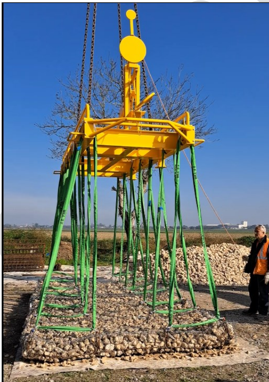
Figure 3: The lifting frame operating with a RenoMac Plus unit before (left) and after (right) releasing the hooks
