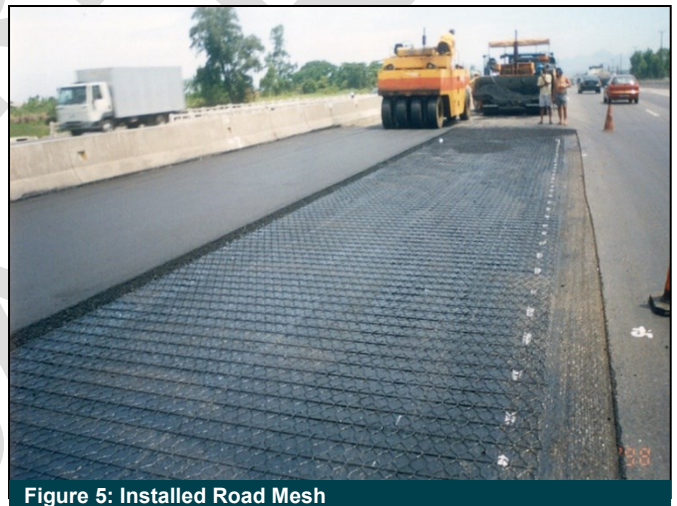
Figure 5: Installed Road Mesh
