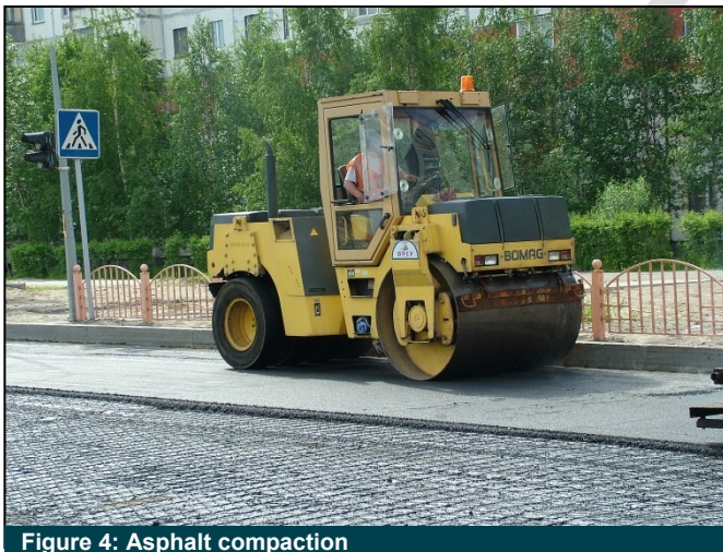
Figure 4: Asphalt compaction
