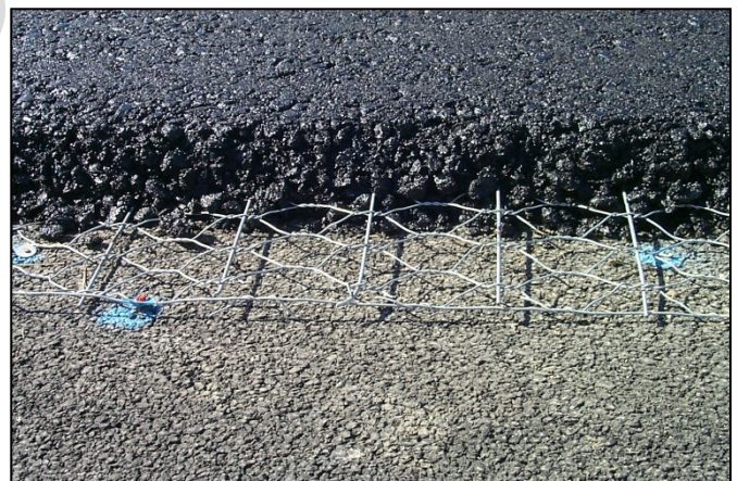
Figure 3: Road Mesh reinforces the asphalt layers
