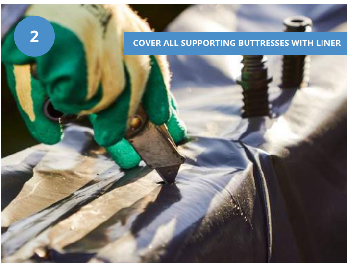
Get your liner into position - make small incisions for the final layer dowels to push through the liner.
