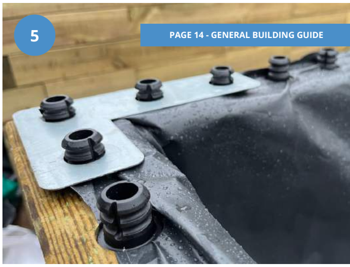
Install your angle corner plates - use your dowel protector to hammer these plates firmly into place.
