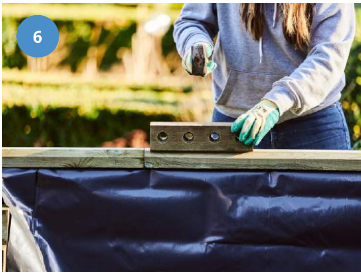
Knock on your capping layer - use a spare BlocX to protect the wood when hammering. JOB DONE!
