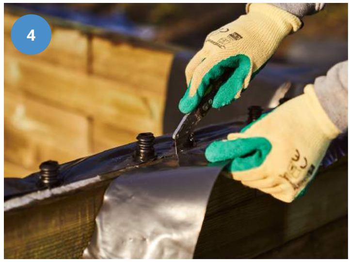
Trim excess liner with a sharp knife - using a retractable blade carefully cut away overhanging liner.
