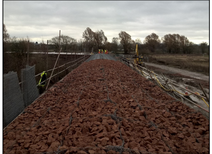
Reno mattress 230mm thick filled with local 6G stone
