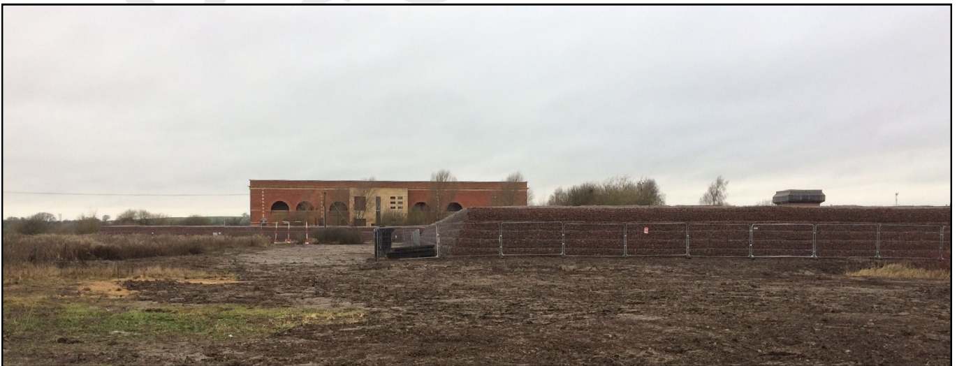
View of the external side of the completed repair works - Feb 2017
