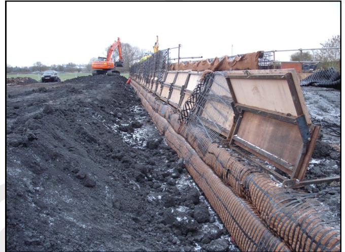
Flood protection bund during construction in 2010/11
