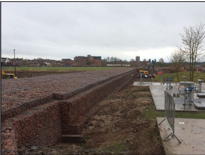
Internal side - Project completed Feb 2017
