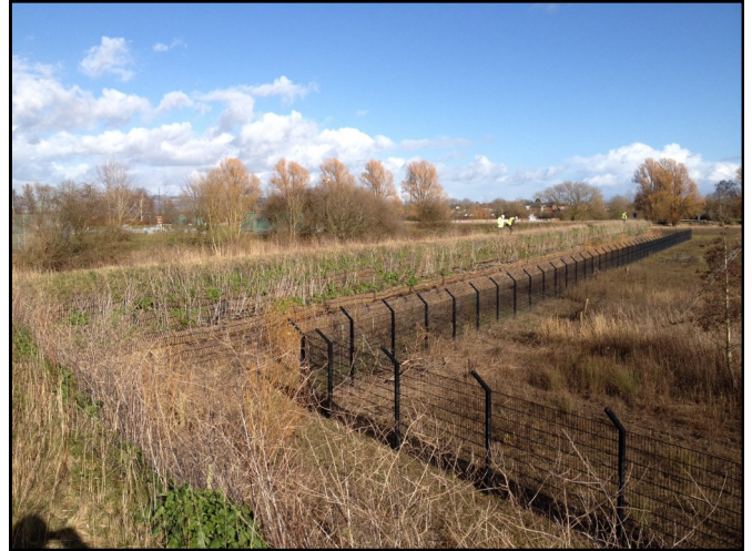
Existing structure before the repair works
