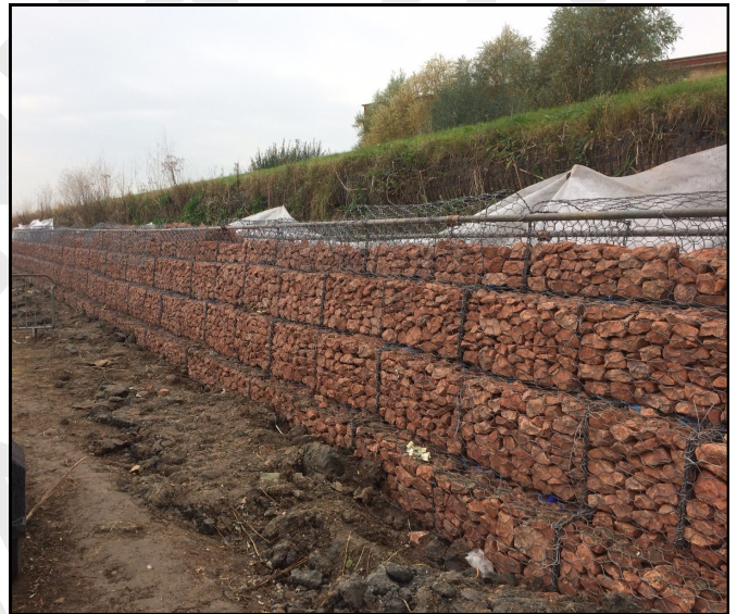
External side of the structure during construction - Nov 2016
