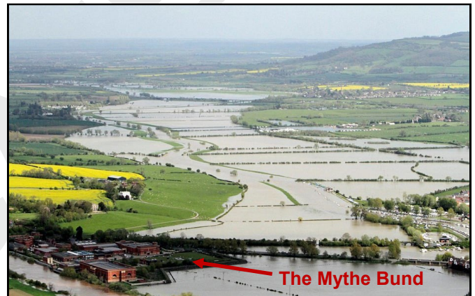
April 2012 - Flood in Tewkesbury
