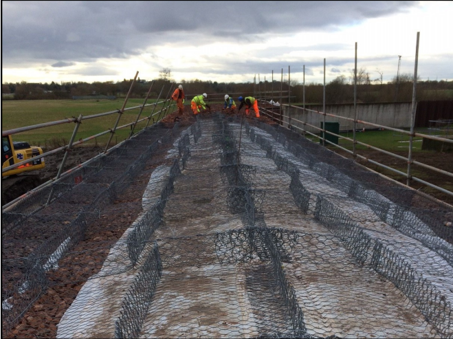
Reno mattress placed over the top of the bund
