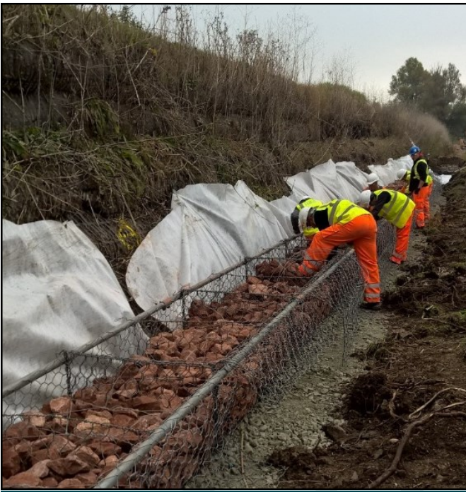
Maccaferri Construction on initial phases - Oct 2016
