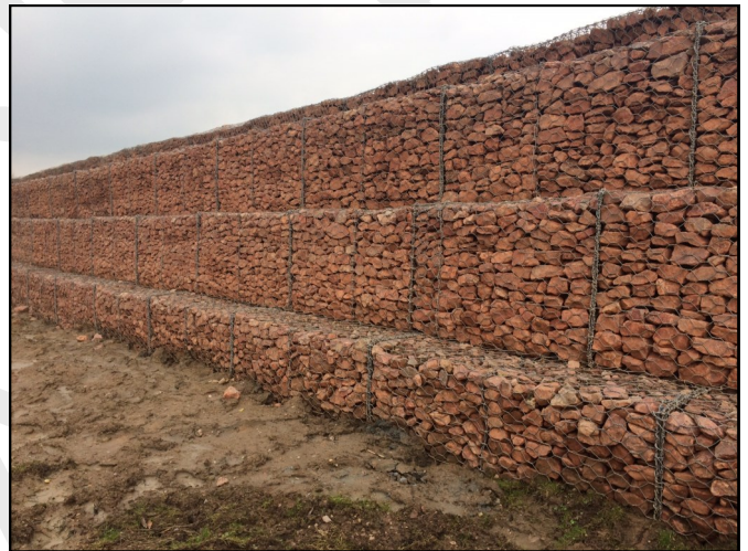
Internal side - Project completed Feb 2017
