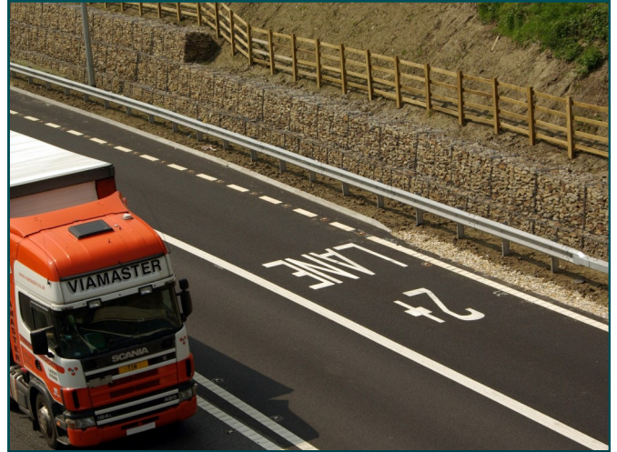
Post-construction - East bound
