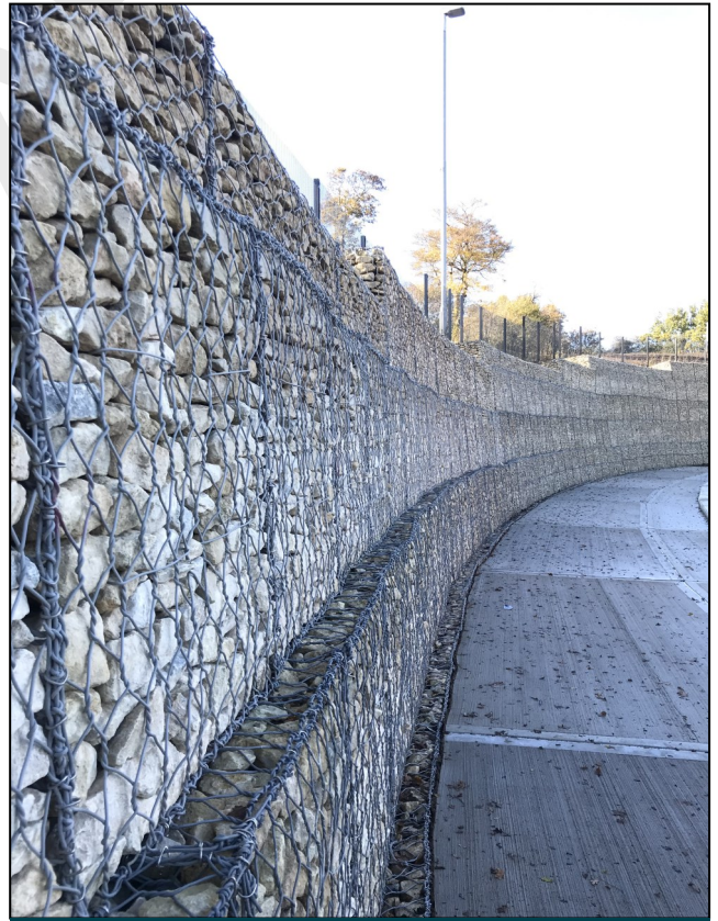
Close up of the wall with the DT mesh
