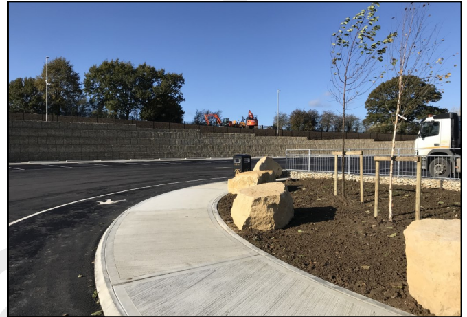
The tallest part of the wall at 5.5m high
