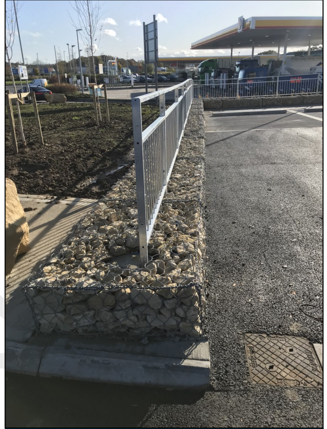
Stand alone gabions with safety rails
