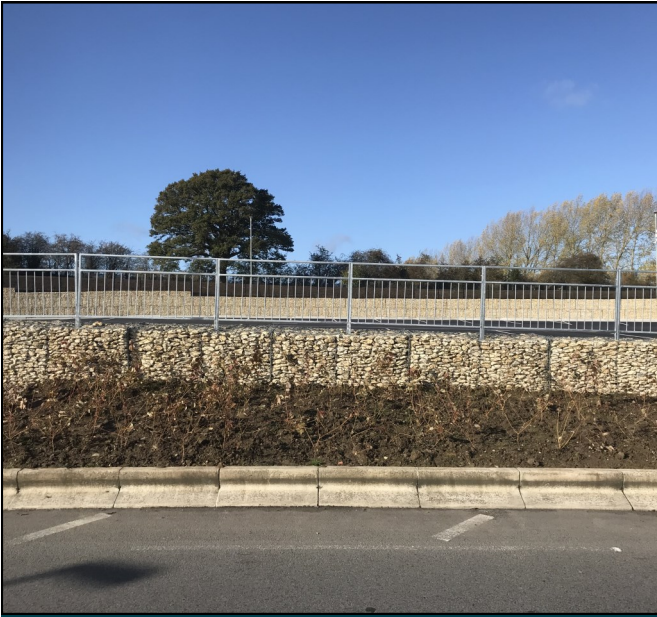
Gabions with rail inserted planted trees & shrubs in front
