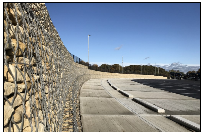
Terramesh wall runs to edge of parking area and steps down
