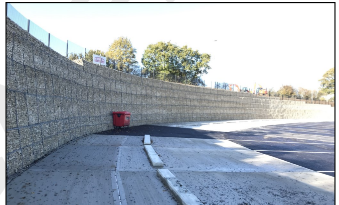
Neatly placed stone in the gabions minimising voids
