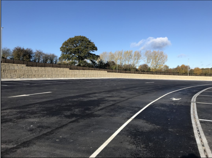
The wall surrounding the slip road and then the HGV parking area
