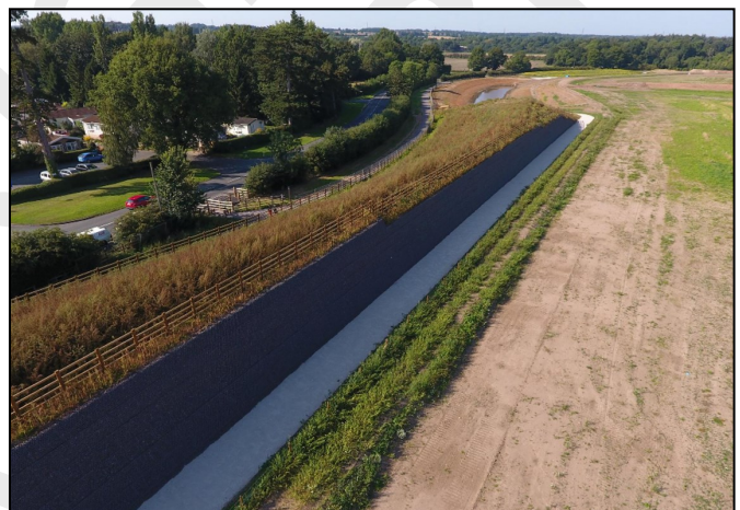
Completed Mineral Terramesh structure **
