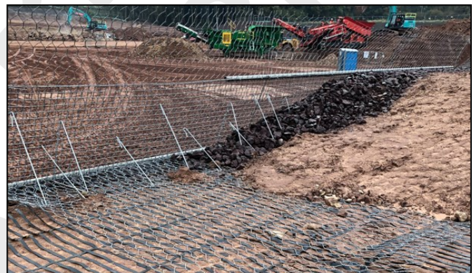
Mineral Terramesh bracing rods installed
