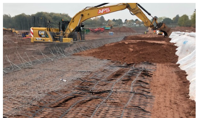
Site won class 1A fill being placed on ParaGrid reinforcement
