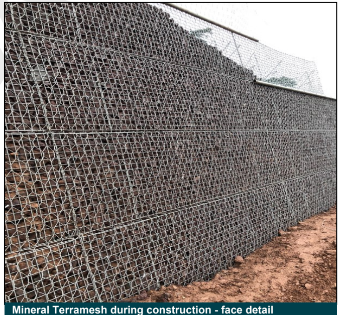
Mineral Terramesh during construction - face detail
