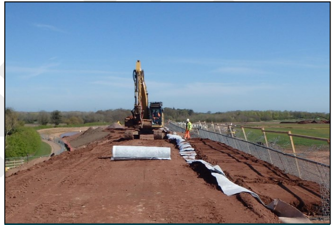
MacDrain geocomposite installed **
