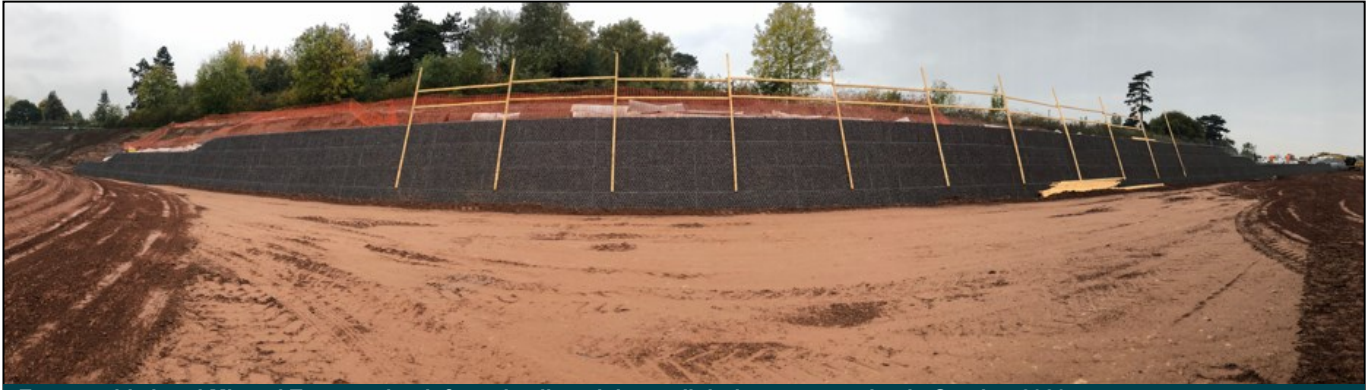
Eastern side bund Mineral Terramesh reinforced soil retaining wall during construction in October 2020
