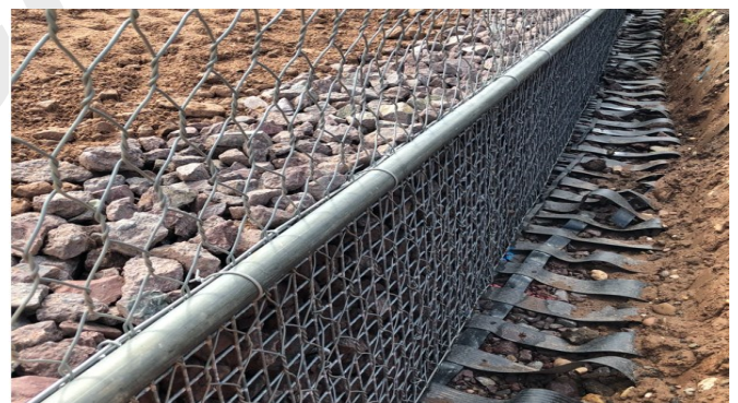
Low height western boundary wall being constructed
