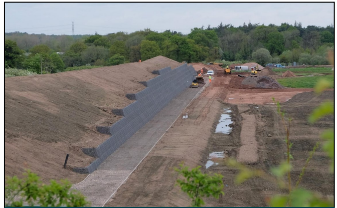
Structure reaching full height **
