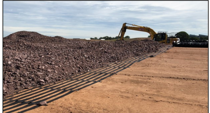
ParaLink basal reinforcement being installed
