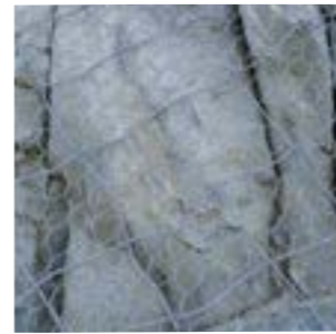
3 Mesh Systems - Secured Drapery / Surface Stabilisation
