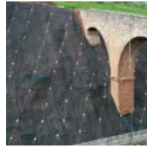
6 Soil Nailing and Surface Protection
