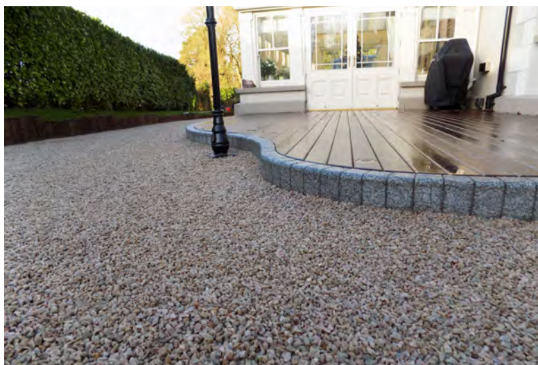
▲ Private Drive (above) & Garden (below) - Irish Barley Quartzite Aggregate
