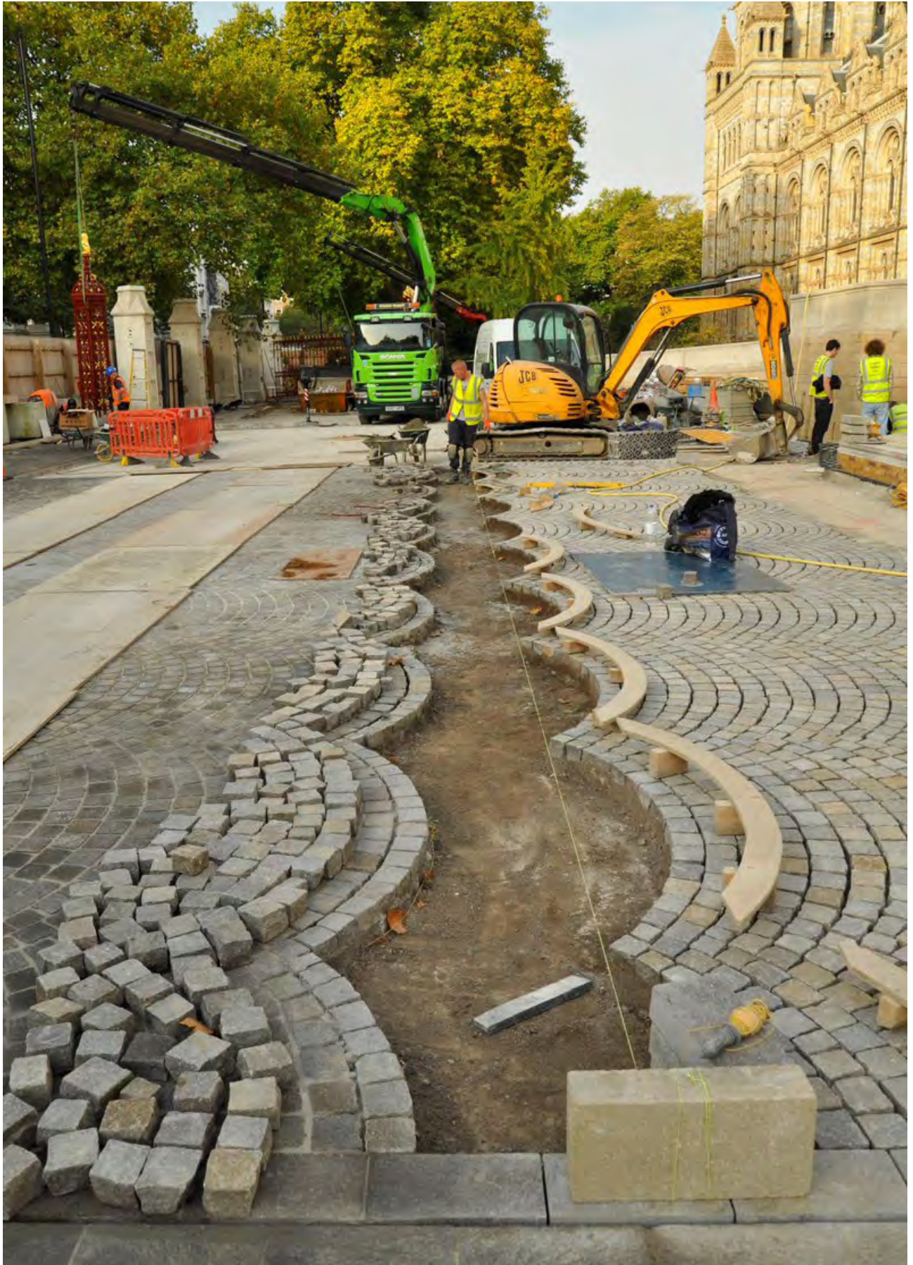
▲ Porphyry Setts being laid at Natural History Museum.
