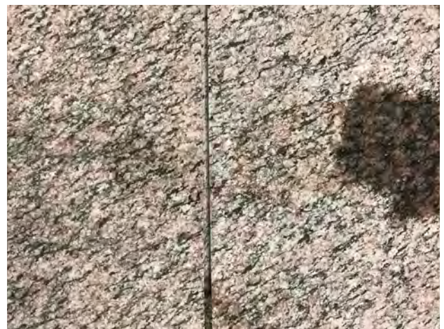
The area has been thoroughly cleaned off using water.
