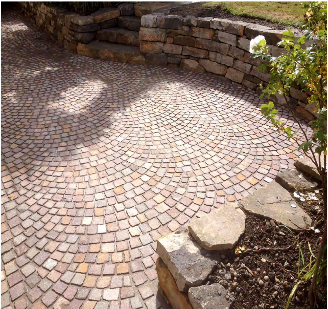
▲ Contractor: Gray Stoneworks - Products: Italian Porphyry Setts
