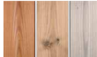
At Installation 6 months + 1 Year +
