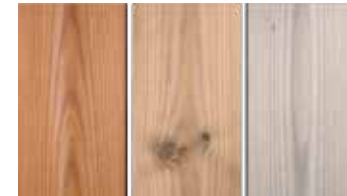
At Installation 6 months + 1 Year +
