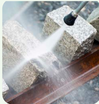
Step 2 Clean paving and base
