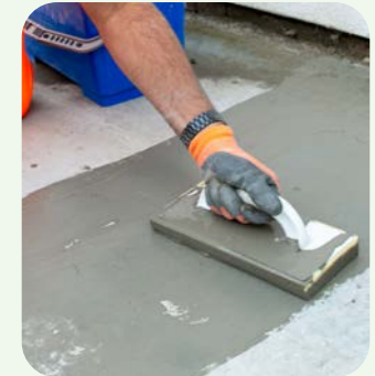
Step 6 Apply bonding mortar to base
