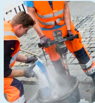
Step 4 Add tufftop and mix together
