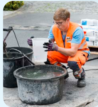
Step 3 Add water to a bucket or mixer
