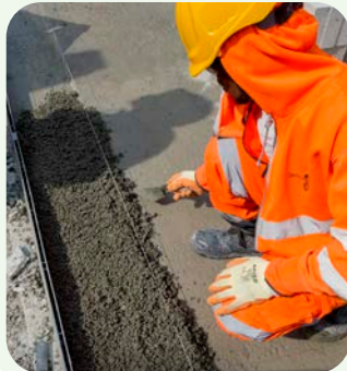
Step 7 Place the tuffbed 2-pack
