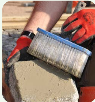
Step 8 Brush on the bonding mortar
