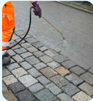
Step 2 Wash and wet paving
