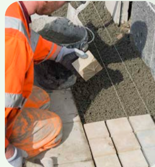
Step 9 Tap unit down to level
