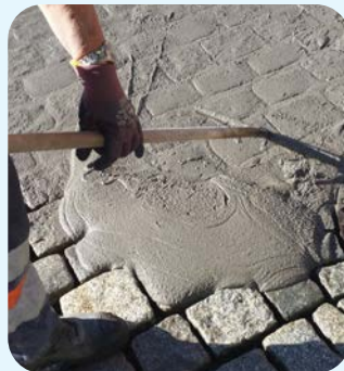
Step 6 Spread into joints
