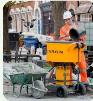
Step 3 Add the aggregate
