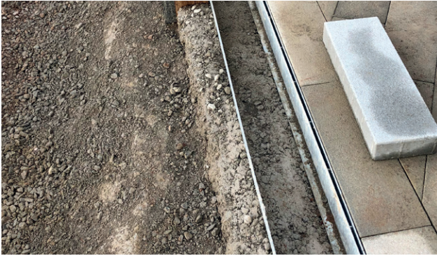
Installation of ACO Qmax slot drainage
